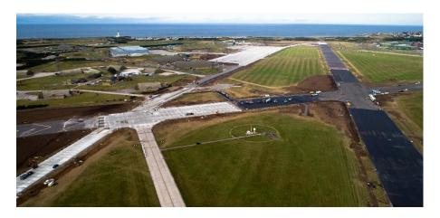
In September 2023, a significant schedule of works began at RAF Leeming. The Airfield Refurbishment project will provide serviceable operating surfaces via a scheduled rehabilitation of the existing pavements and lighting to ensure that existing operations are maintained.
